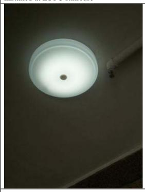
iLighting Supplies sensor controlled 10W LED Circular lamp to replace 22W FL lamp at Staircase of Peak Tower HK for Hang Lung Real Estate Management to demonstrate the energy saving through lighting retrofit by LED with intelligent sensor control.
